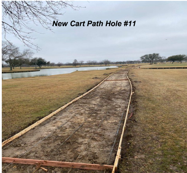
Forms for Cart Path Installed
